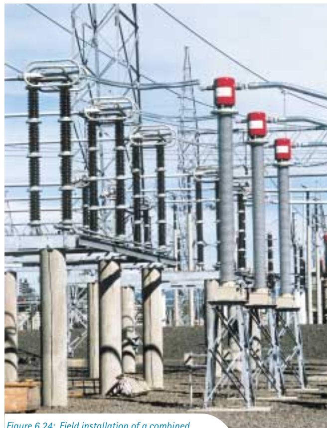
Figure 6.24: Field installation of a combined optical CT/VT
